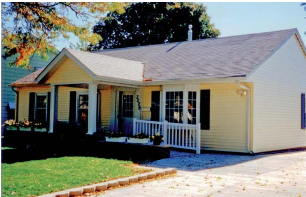
An addition need not be large to have a big impact, such as the home featured above, which has added a better ramp, wider door and weather-protecting overhang on the front porch.
