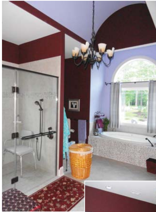
A curbless shower and adjustable hand-held controls allow John to use the spacious master bathroom. INSET: The master bath’s sink area has open knee space at both stations.
