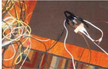
Old plug adapters and old cords piled on top of each other can overload, overheat and start a fire.
