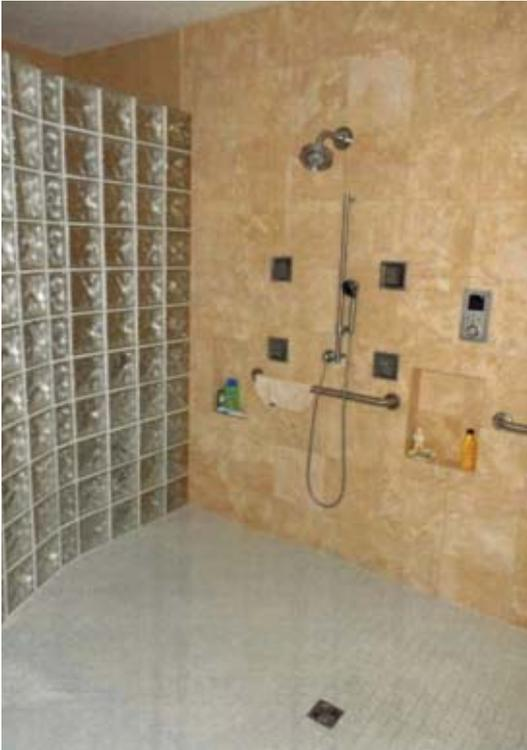
This “wet room” is designed with additional floor drains and moisture venting.
