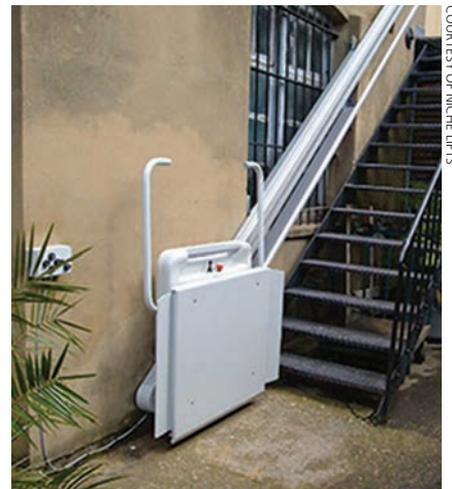
An incline lift, shown in folded position.
