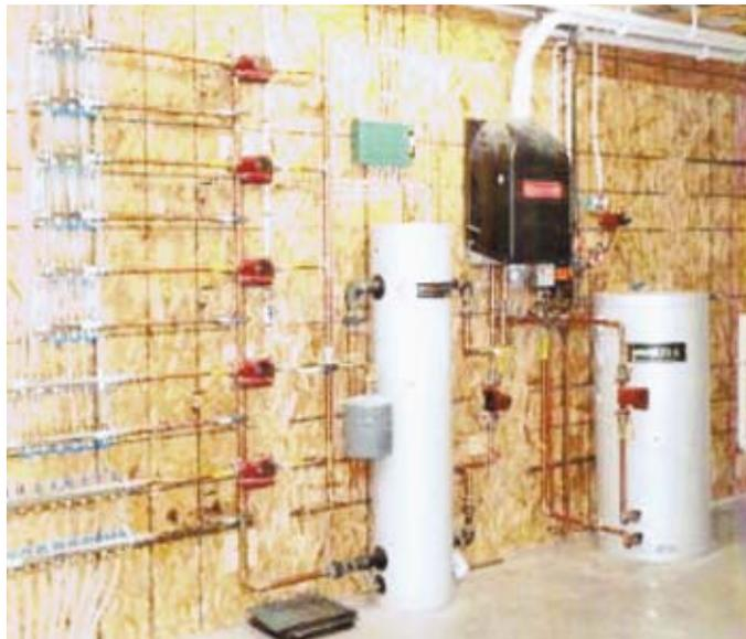
Geothermal ground heat provides hot water for in-floor radiant heat. Photo shows water-holding tanks and manifolds to disperse water to separate zones.
