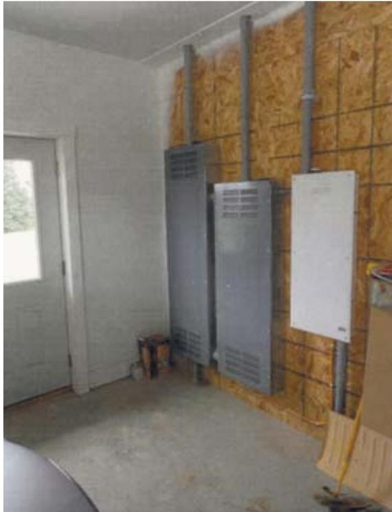
Geothermal and electrical panels are at an accessible height (no more than 48 inches to the highest switch) and in an accessible location.
